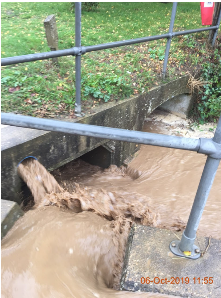
Entry to culvert at junction of Grove Road and Church Path
